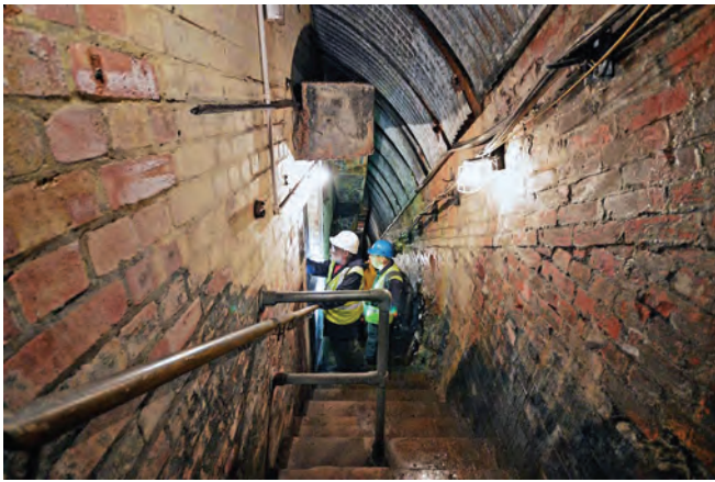
SubBrit member Mike Stace looking into the BBC Transmitter Room
